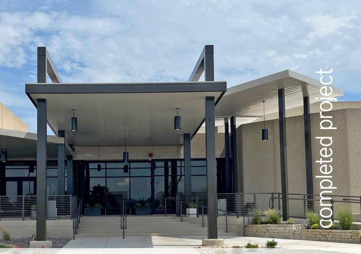
Our HSS tube steel canopies are meticulously crafted, to reduce bird nesting ledges, enable hidden bolts and allow for internally-routed conduit. Finished parts receive a Poli-5000 powder coat finish for a sleek look, all backed by a 10-year warranty.
